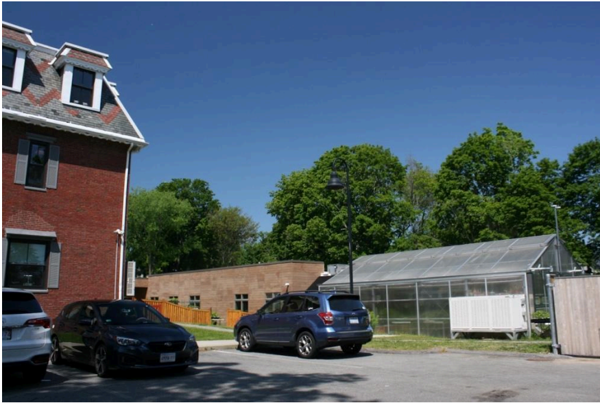
Figure 18. South elevations of new additions on the north side of the property. The east elevation of the 1859 building is on the far left. Photograph by Wendy Frontiero, June 2023.
