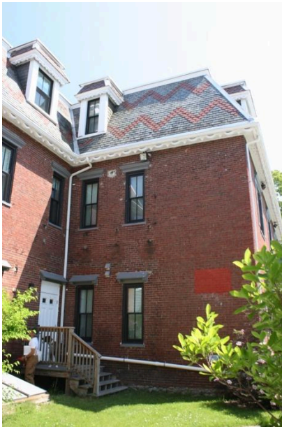
Figure 7. West elevation of the main block. Photograph by Wendy Frontiero, June 2023.
