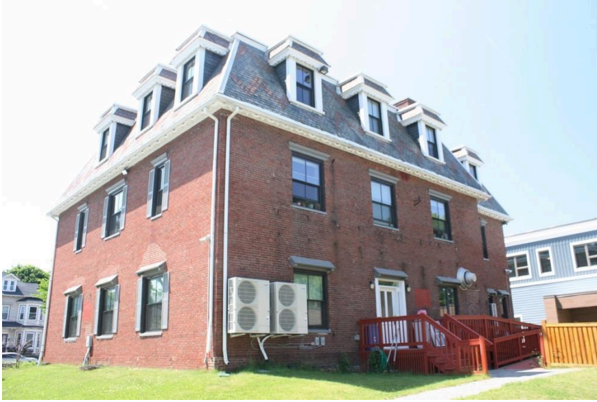
Figure 10. East and north elevations. Photograph by Wendy Frontiero, June 2023.
