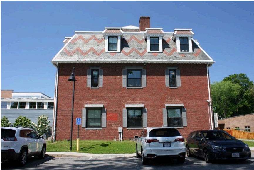
Figure 11. East elevation. Photograph by Wendy Frontiero, June 2023.
