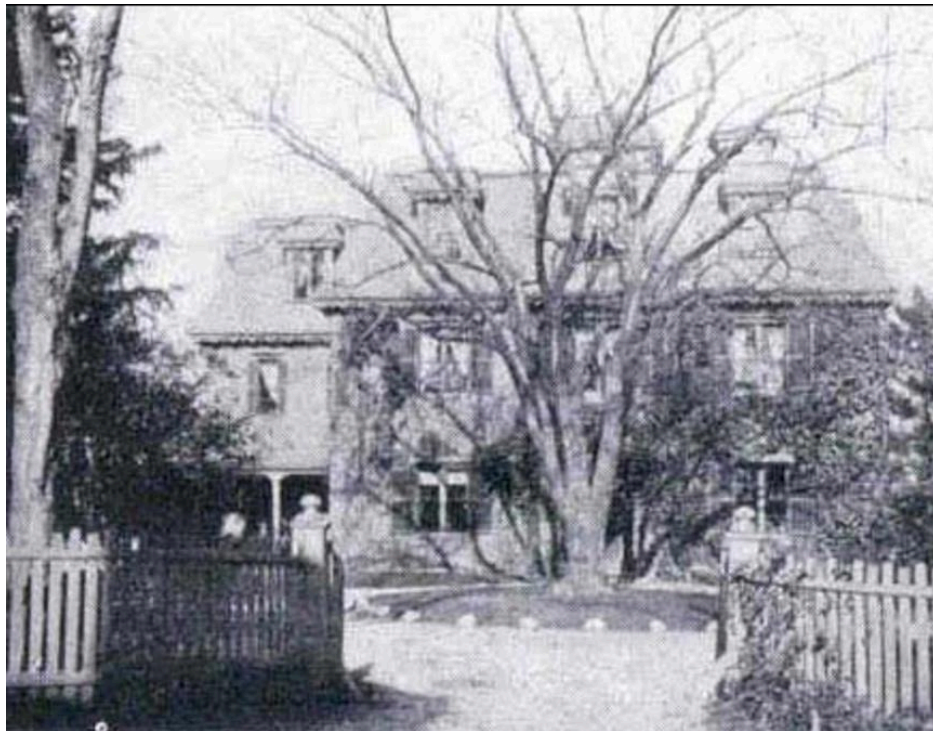
Figure 22. View of façade ca. 1898, looking north.
