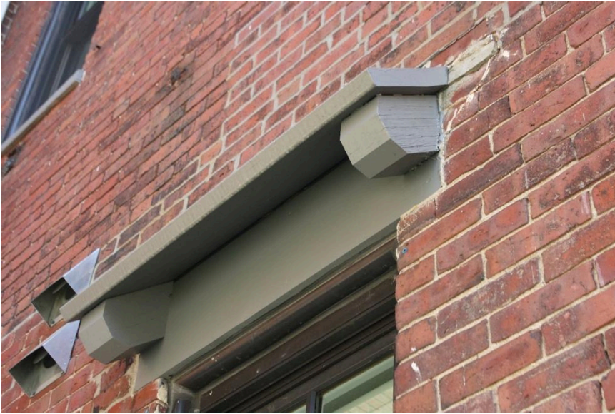
Figure 12. Detail of typical window and door trim. Photograph by Wendy Frontiero, June 2023.
