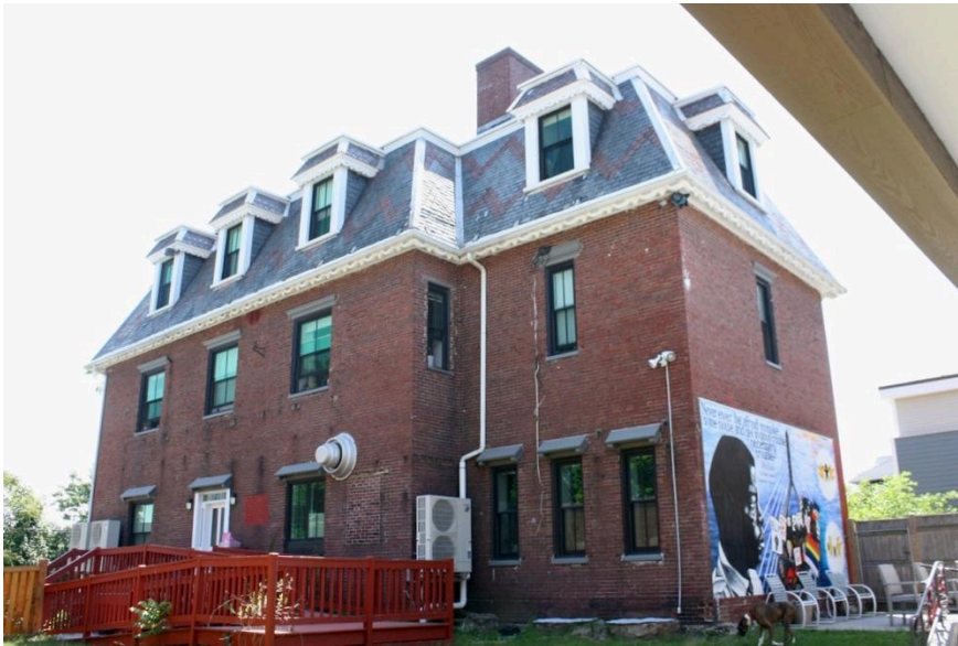
Figure 9. North and west elevations. Photograph by Wendy Frontiero, June 2023.
