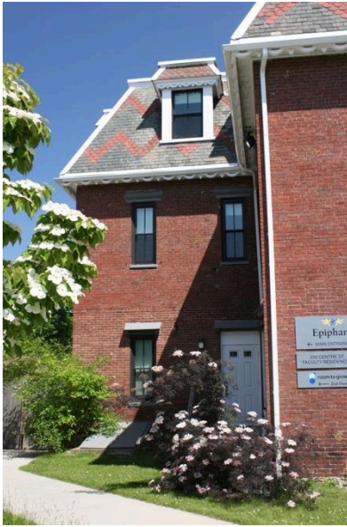
Figure 8. Façade (south elevation) of kitchen wing. Photograph by Wendy Frontiero, June 2023.
