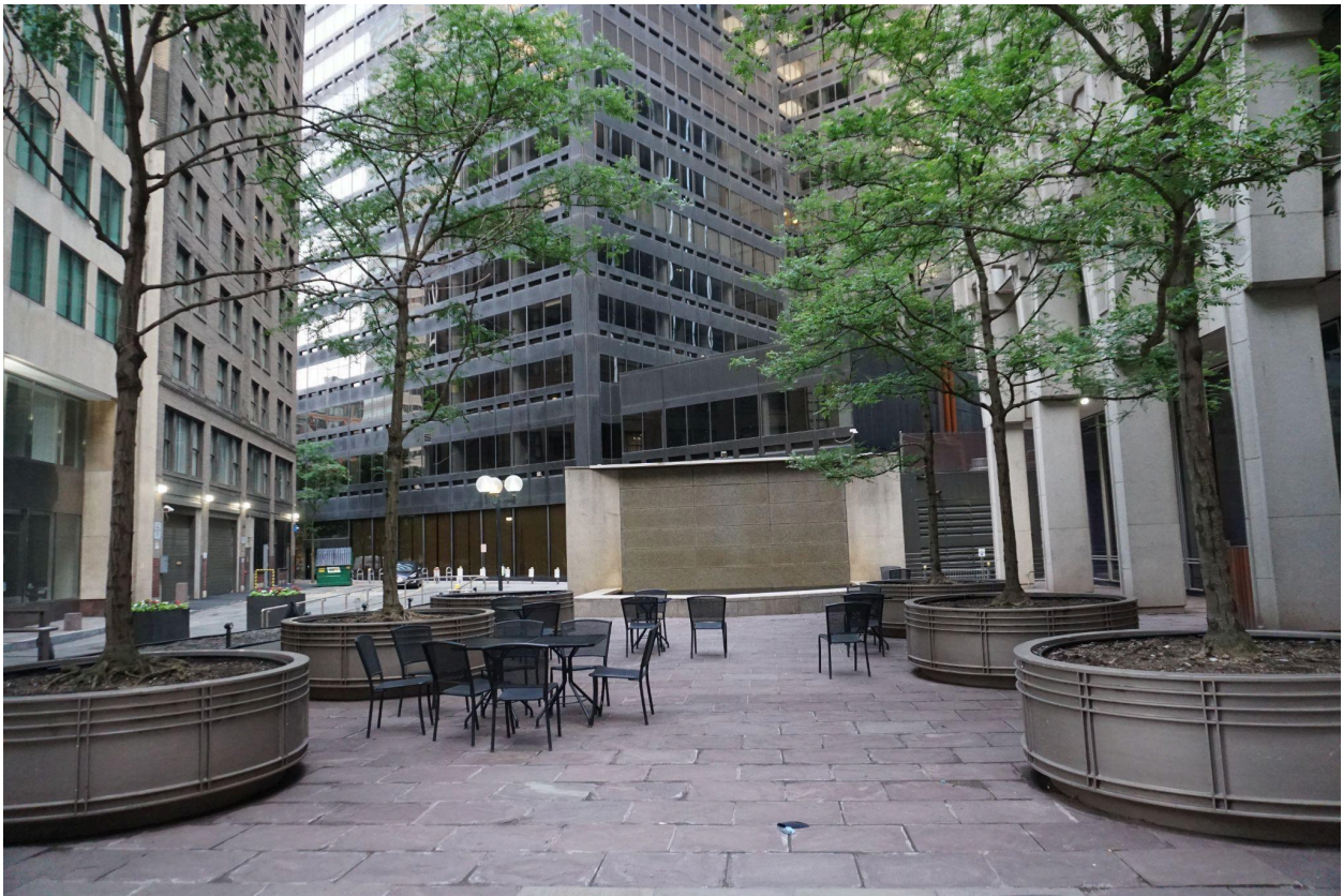
Figure 8. Plaza with round planters (which replaced original pyramidal skylights) and fountain wall in background, looking west, June 2023. Photo credit: Building Conservation Associates.
