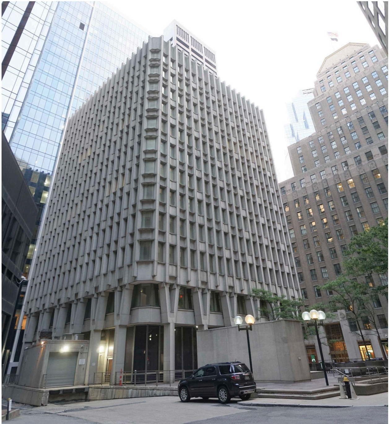
Figure 4. South and west elevations, June 2023. Photo by Building Conservation Associates.
