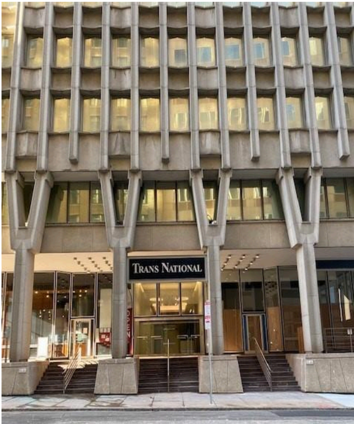
Figure 6. East entrance, January 2024. Photo by BE Realty.
