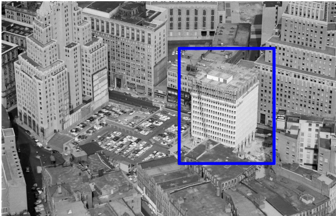
Figure 14. Blue Cross building under construction, Financial District, Boston, 1958-1960.
