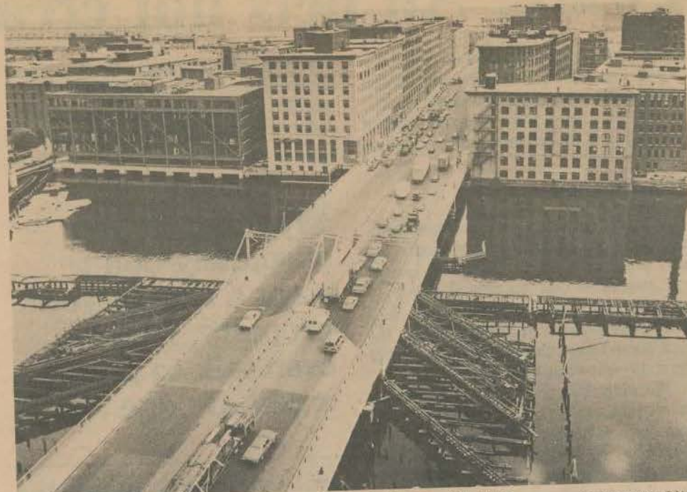
The Summer Street Bridge: Tracks for the old drawbridge are still visible.
