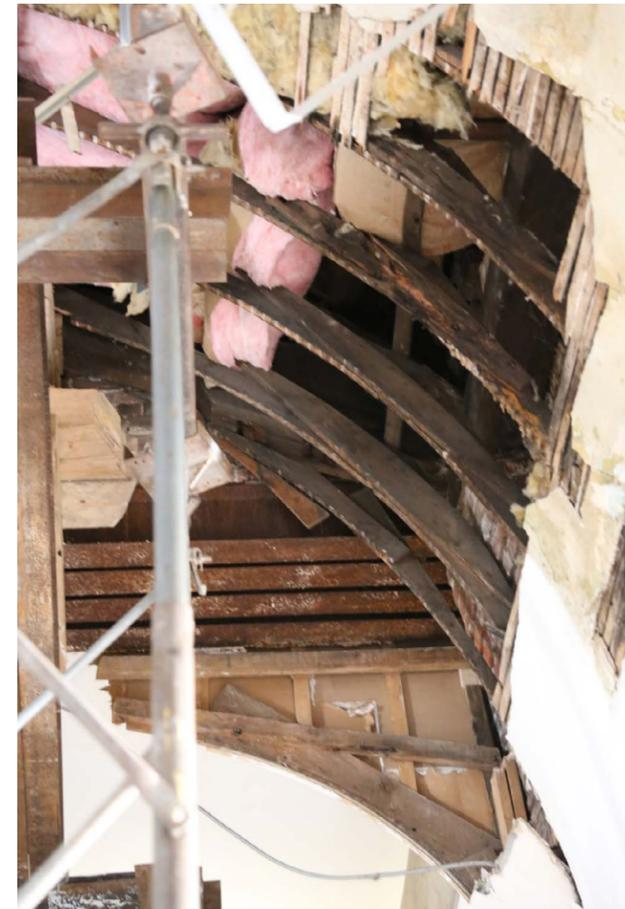
Probes and Shoring at roof framing (Spring 2019)
