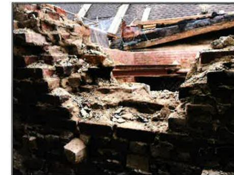
Ultimately, Gale's opinion was developed that the demolition method was not positively correlated to the poor bond strength discovered to exist throughout the wall. It was Gale's conclusion that the condition of the tower masonry walls, at the current level of demolition, would be incapable of supporting the weight of a new belfry and spire and recommended stabilization methods for the remaining tower structure could be extensive and, as such, possibly not cost effective.
