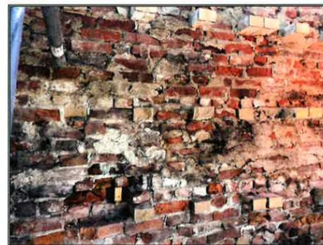
At many locations, inner red brick wythes could be removed by hand and were found to have little mortar bond between courses.
