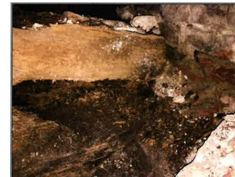
Additionally, adjacent to the truss, a portion of the structural steel lintel supporting the entire weight of the remaining east tower masonry wall was observed to be severely deteriorated. The visible portion of the flanges and web of the lintel was observed to have significant section loss, including a hole through the web at its end.
