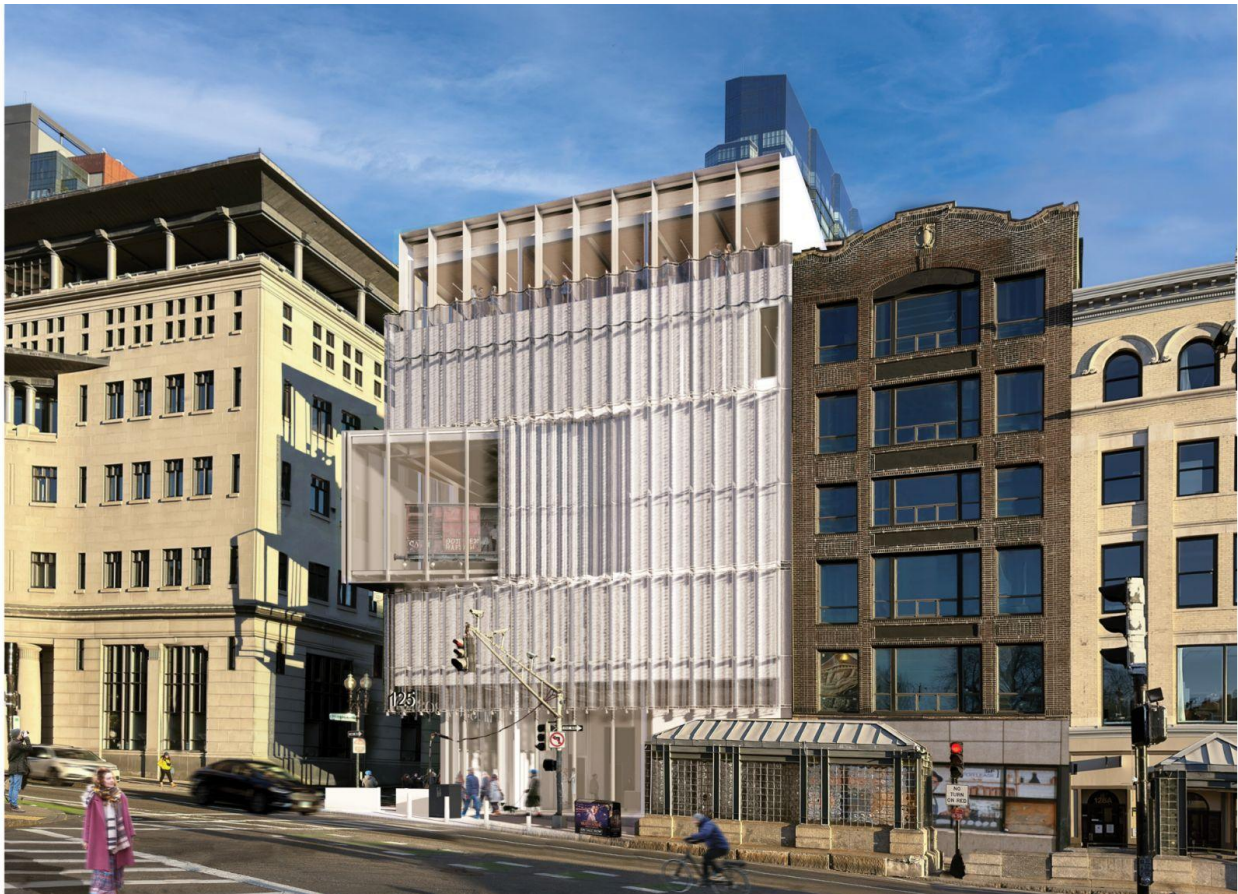
Figure 9-12 Exterior View - From the Boston Common
