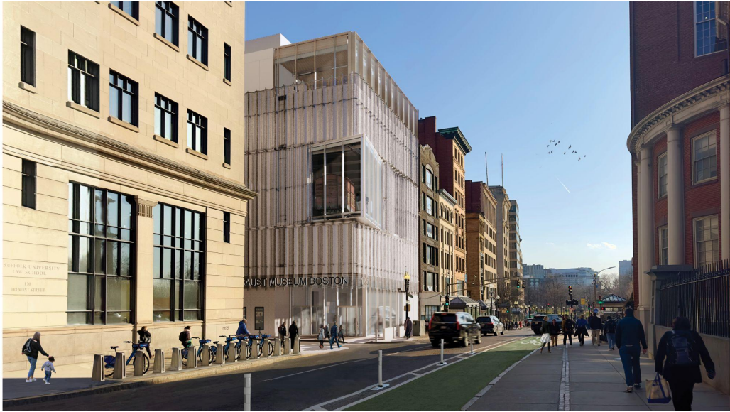
Figure 9-10 Exterior View - From Tremont Street
