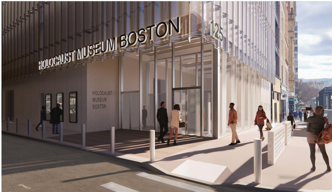
Figure 9-9 Exterior View - Entry at Tremont Street
