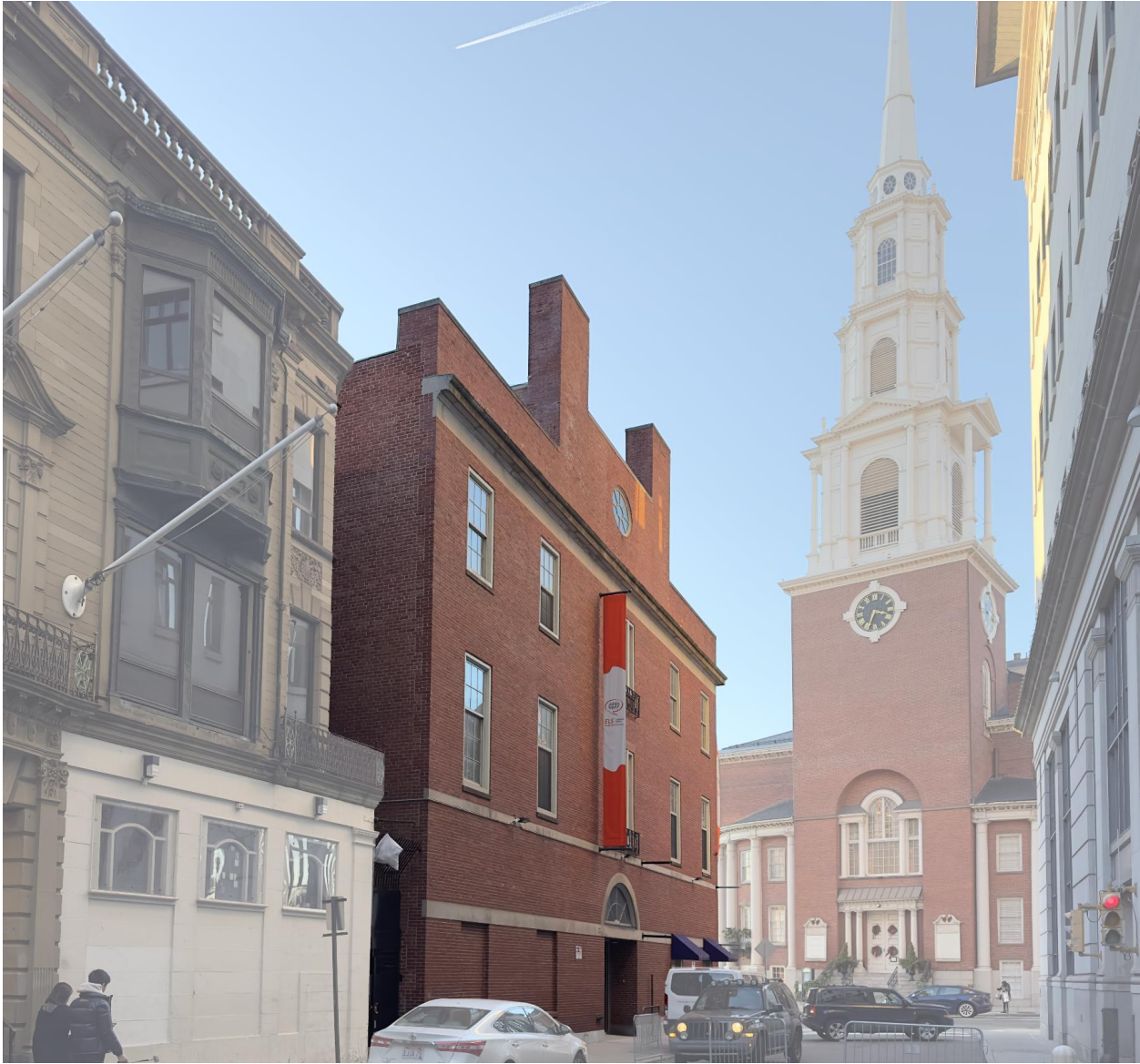
Figure 4-3 Site View from Hamilton Place, 125 Tremont Street, Boston, MA
