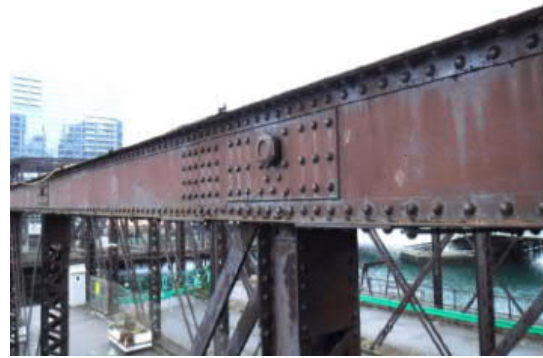
Image 4: Typical Top Chord Member in the Approach Spans
