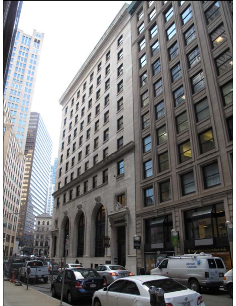
Devonshire St. facade, view from northeast.
