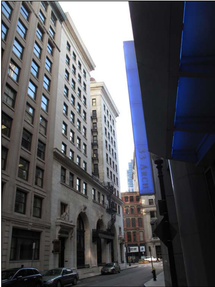
Arch St. facade, view from northwest.
