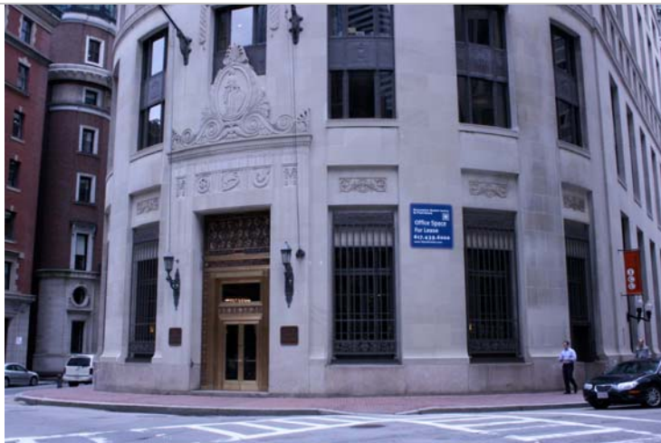
Ground floor detail – Liberty Square
