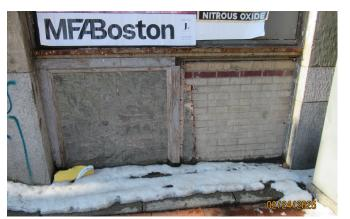
D. EXIST BRICK INFILL AT BASEMENT WINDOWS WITH TRUE EXTERIOR BOARD AND TRIM TO RECREATE RECESSED
